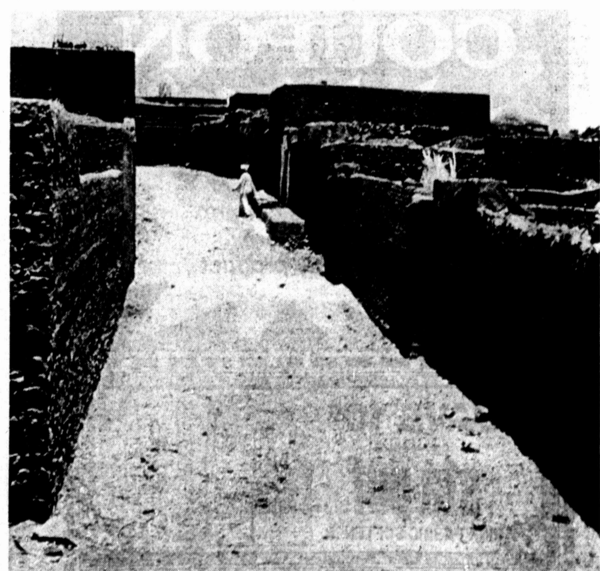
DESIGNED FOR CLIMATE — A small Egyptian village along the Nile River features homes that were built without roofs. In some areas of Egypt, several years can pass without measurable precipitation.
