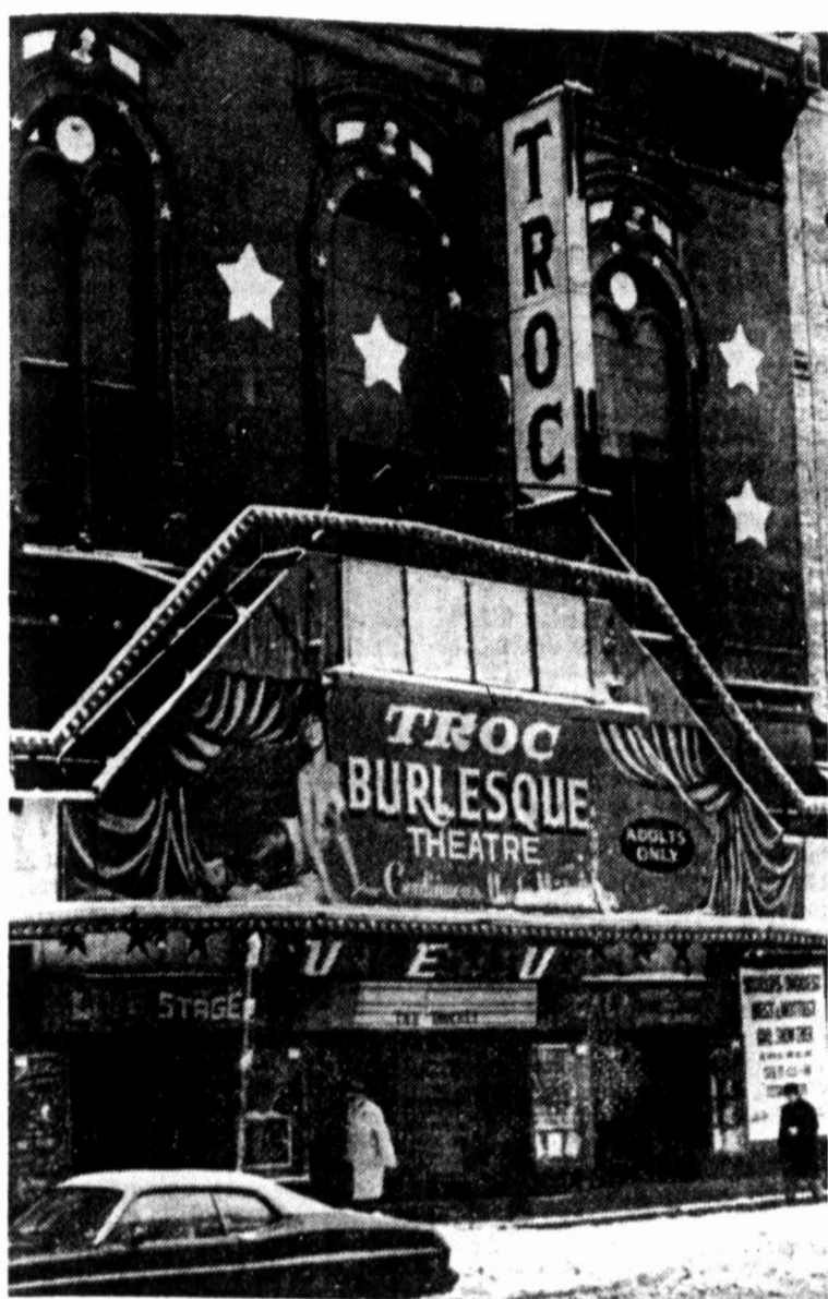
TO BE CHINESE THEATER — The Troc Burlesque Theatre will not be a place for striptease girlie shows after March 31 when remodeling will be completed, converting the 75-year-old Philadelphia landmark into a theater for Chinese language movie films (AP Laserphoto).
