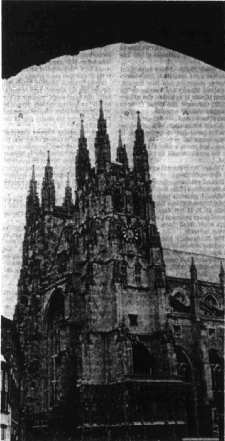
SPIRES AND ARCHES — Built in the 8th century, much of the stone walls and original gates of Canterbury Cathedral still stand.
