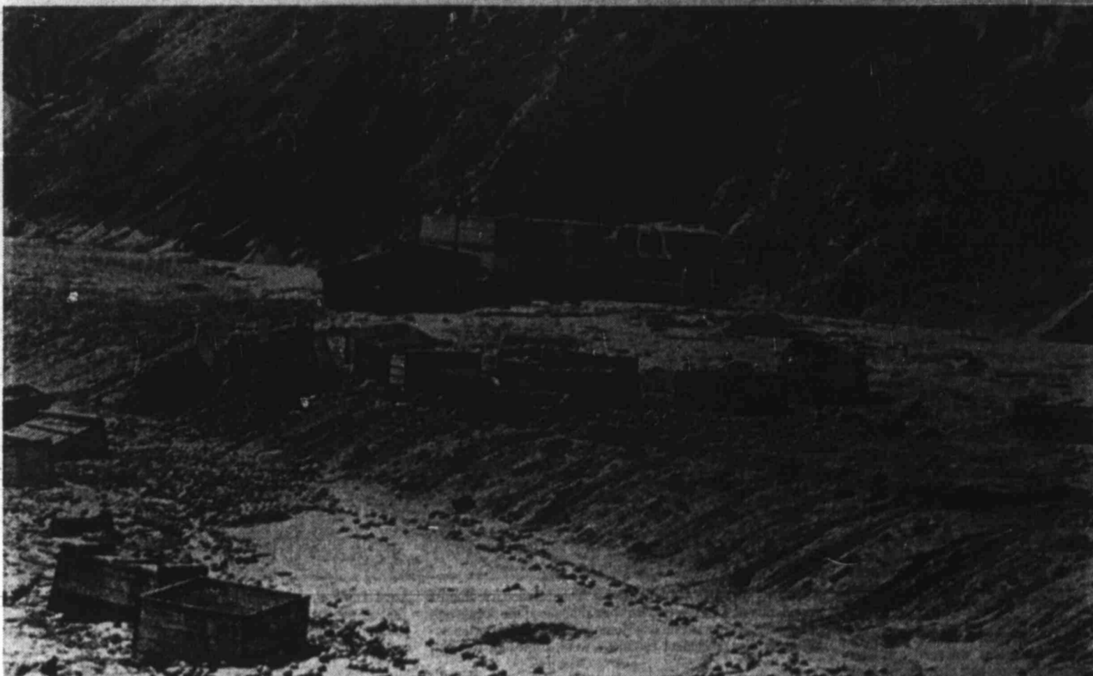
INTERSTATE HIGHWAY BLOCKED BY SLIDE — Southbound lanes of highway Interstate 5 are covered with mud and littered with oranges from a trailer truck shown caught in the mud that came down Sunday near Lebec, Calif. The mudslide, three to
