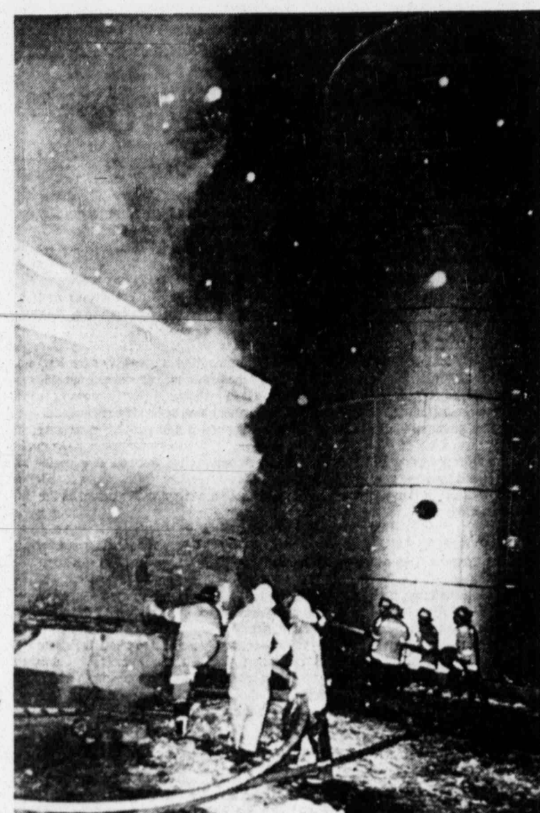
GRAIN ELEVATOR EXPLOSION — Firemen battle a blaze at a feed company near Liberty, Mo., Thursday night after an explosion killed three workers and injured a half-dozen others. (AP Laserphoto)
