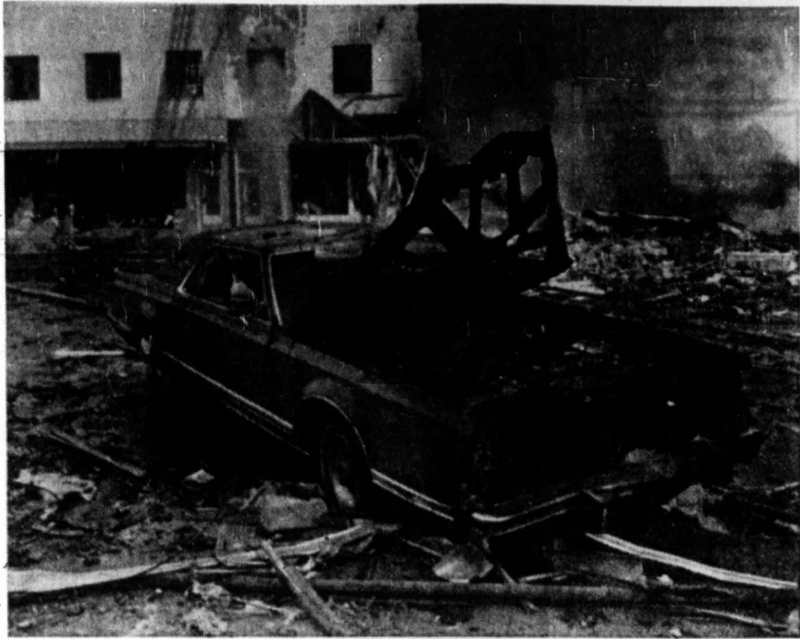
BLAST SCENE — An automobile parked across the street from the scene of a natural gas explosion in downtown Auburn Sunday morning is pictured with its tires flat and interior gutted by fire. The explosion destroyed several buildings and damaged more than 40. (AP Laserphoto)
