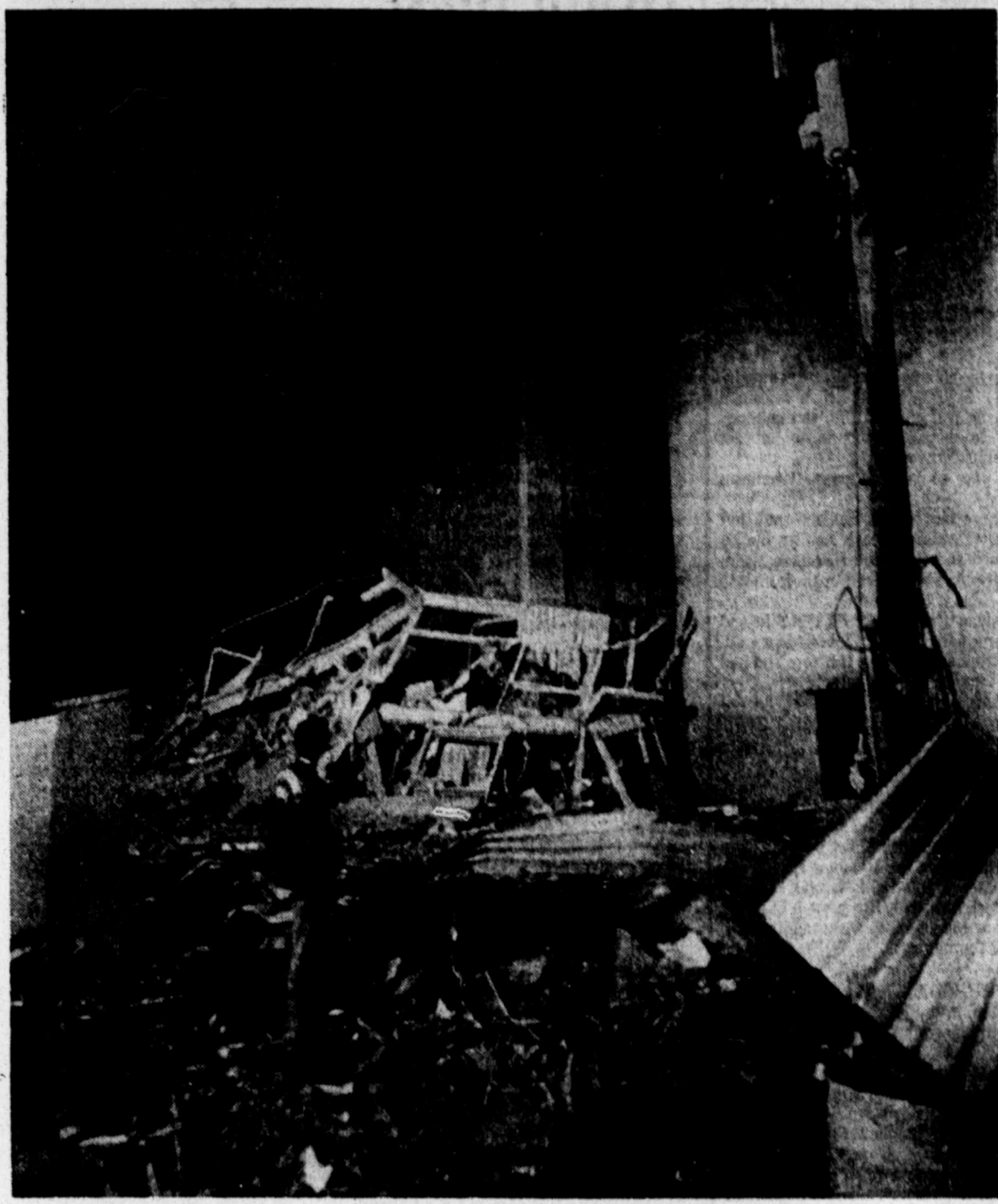
GRAIN ELEVATOR RUBBLE — Concrete and steel combine in twisted wreckage after an explosion ripped through a Galveston grain elevator Tuesday night. At least nine persons were killed in the blast. (AP Laserphoto)
