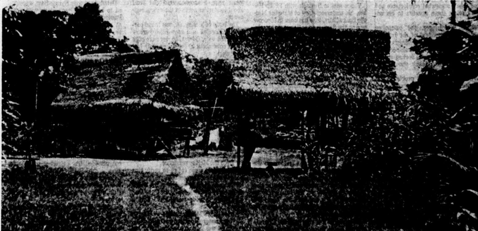
NATIVE CONDOMINIUM — Yagua Indian dwellings, like those of the Jivaro in the same region of the South American jungle, feature open sides. Near Iquitos, tributaries of the Amazon River can rise 20 to 25 feet, so many structures are built on stilts for safety even on high ground.
