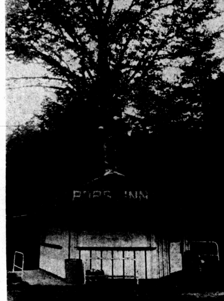
DRIVE-IN TREE — When builders began work on this refreshment stand at Carnation, Wash., years ago, they built around a tree instead of cutting it down. Owners say the tree is a help — it provides shade during the summer. (AP Laserphoto)
