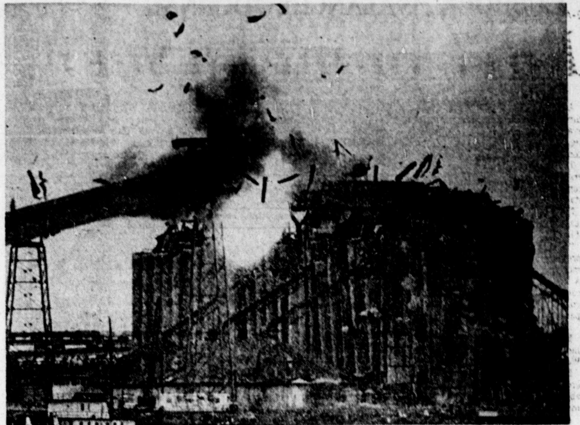
BLASTING — A Conveyor chute for moving grain is blown up at the Continental Grain Elevator near Westwego, La. The chute was blown up to keep it from falling on workers below trying to recover bodies buried by last week's explosions. (AP Laserphoto)
