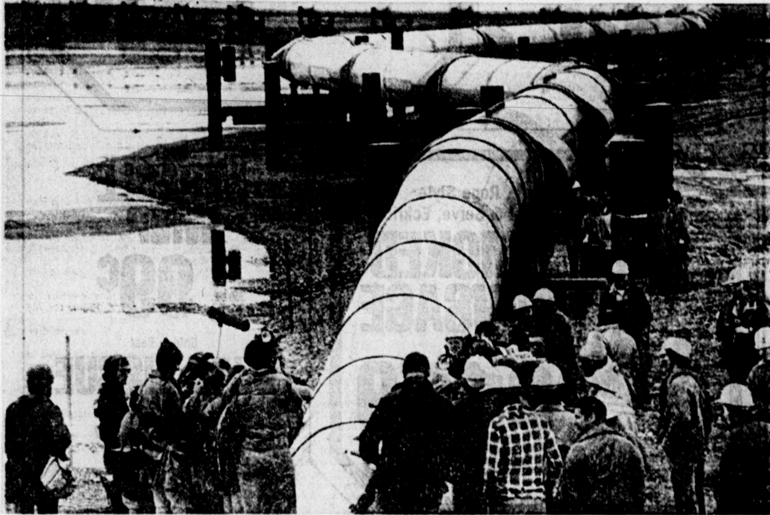
WAITING FOR THE PIG — Newsmen and photographers and pipeline officials waited in this scene at Prudhoe Bay in Alaska last June 21 for the pig, a plug that leads oil down the pipeline, at the exit of the Alyeska oil line pumping station Number One on Alaska's north slope. (AP Laserphoto)
