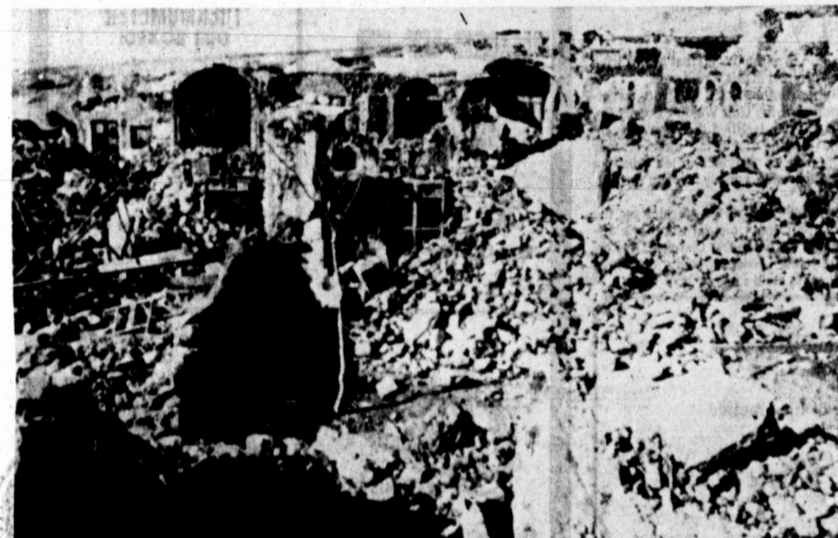
QUAKE TOLL MOUNTS — Rubble fills the ruined streets of village of Sar-Astiyab, Iran Wednesday. The village is one of 16 hard-hit by an earthquake that shook the area 430 miles south of Tehran before dawn Tuesday. Officials said the toll had soared to at least 519 dead and 671 injured in the coal-mining area. (AP Laserphoto)
