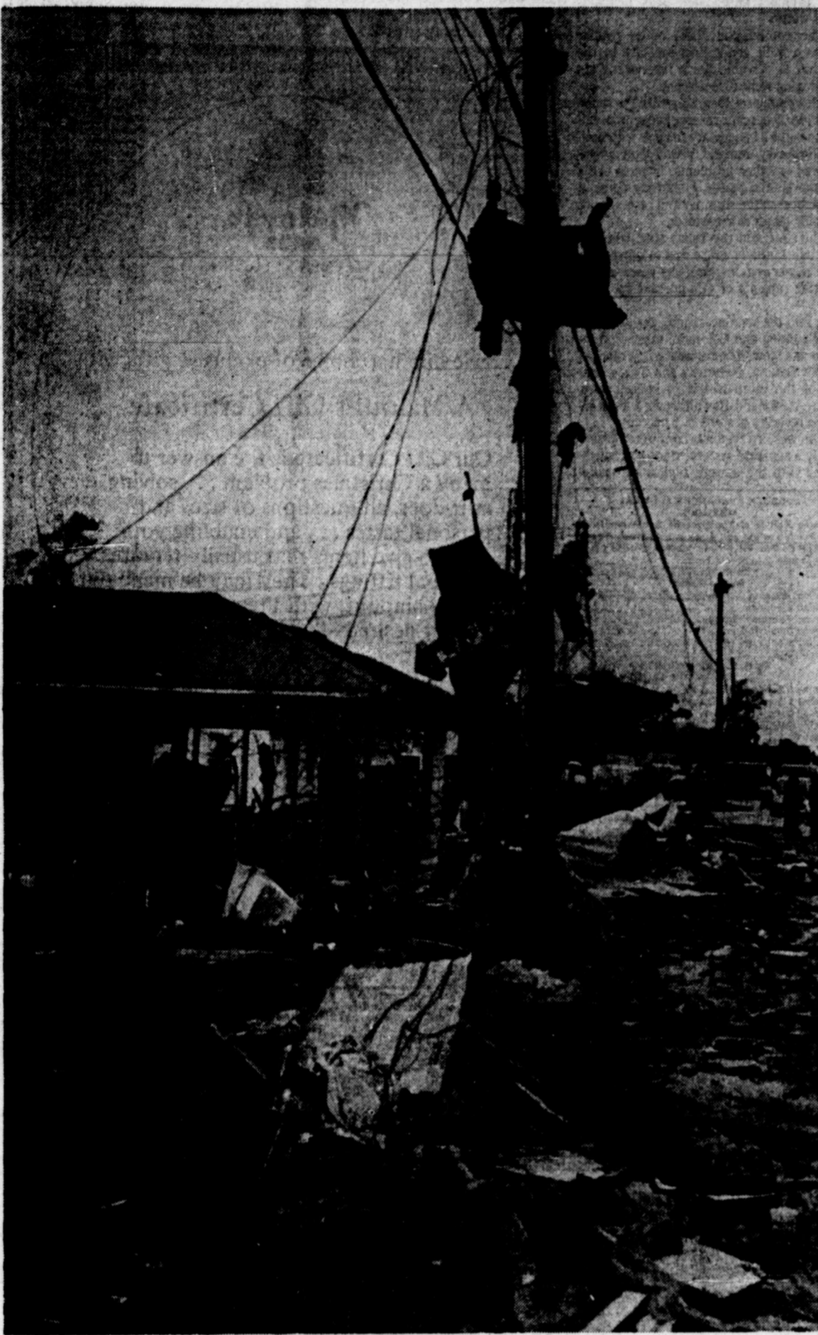
TORNADO PATH —This is the path of a tornado that ripped through the Northeast Houston area Tuesday taking the siding from the building at left and wrapping some of the debris on the power pole. One person was killed by the twister and many others were injured. Additional photos on Page 3, Sec. A. (AP Laserphoto)
