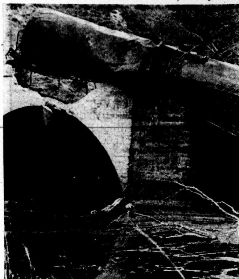
DERAILMENT — These oil tankers, part of 24 cars of the Rock Island Railroad, spilled some oil into Coal Creek near Stuart, Okla., Thursday. Workmen put up an earthen dam to contain the oil. Officials said the tracks collapsed under the loaded train. (AP Laserphoto)
