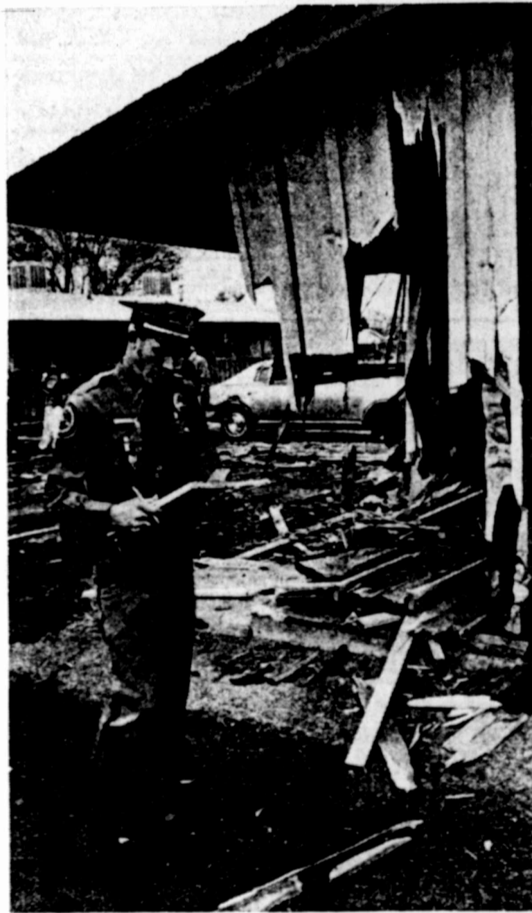
SPLINTERED DEBRIS — A small car driven by a 17-year-old Lubbock youth careened across rain-slicked streets near the intersection of 42nd Street and Avenue L into the side of this apartment complex just as rain began falling over the city Monday. Lubbock patrolman Pat Nesbitt said two occupants of the apartment struck hardest by the vehicle were uninjured, even though they were lying on a couch only feet from where the auto ripped a chunk from the apartment's walls. The vehicle's driver was also uninjured, but police said damage to the complex was "extensive." (Staff Photo by Norm Tindell)
