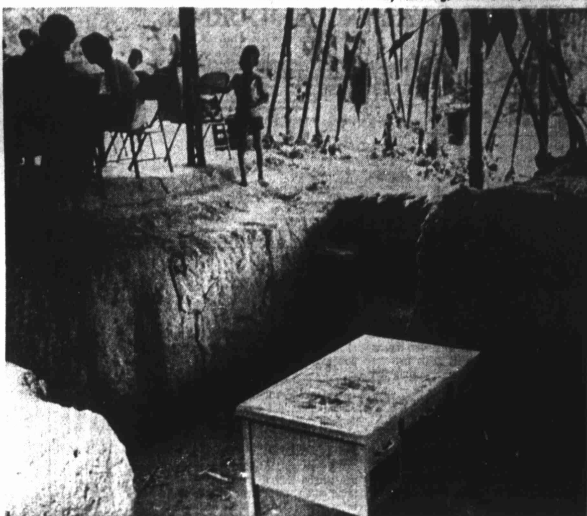
TUNNEL HEADQUARTERS—A single metal desk gives an idea of the scale of the command bunker of the Chu Chi Liberation Battalion near Chu Chi, Vietnam. From this nerve center of an underground tunnel octopus 20 miles northwest of Saigon, Vietnamese units were able to move some 150 miles, sometimes
