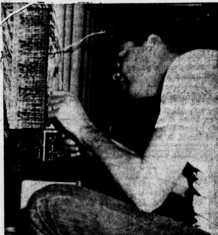
MAKING TELEPHONE PROGRESS - General Telephone Co. is converting its equipment here to modern seven-digit service, and the plant here as a result is undergoing extensive revamping. Here are two scenes in the Muleshoe plant where craftsmen are doing the tedious job of rewiring. At top Joe Lee Robinson is peeling a 600-pair cable, while at the bottom Larry Deering makes one of the multitude of connections which must be made before the system goes into effect late in the summer.
