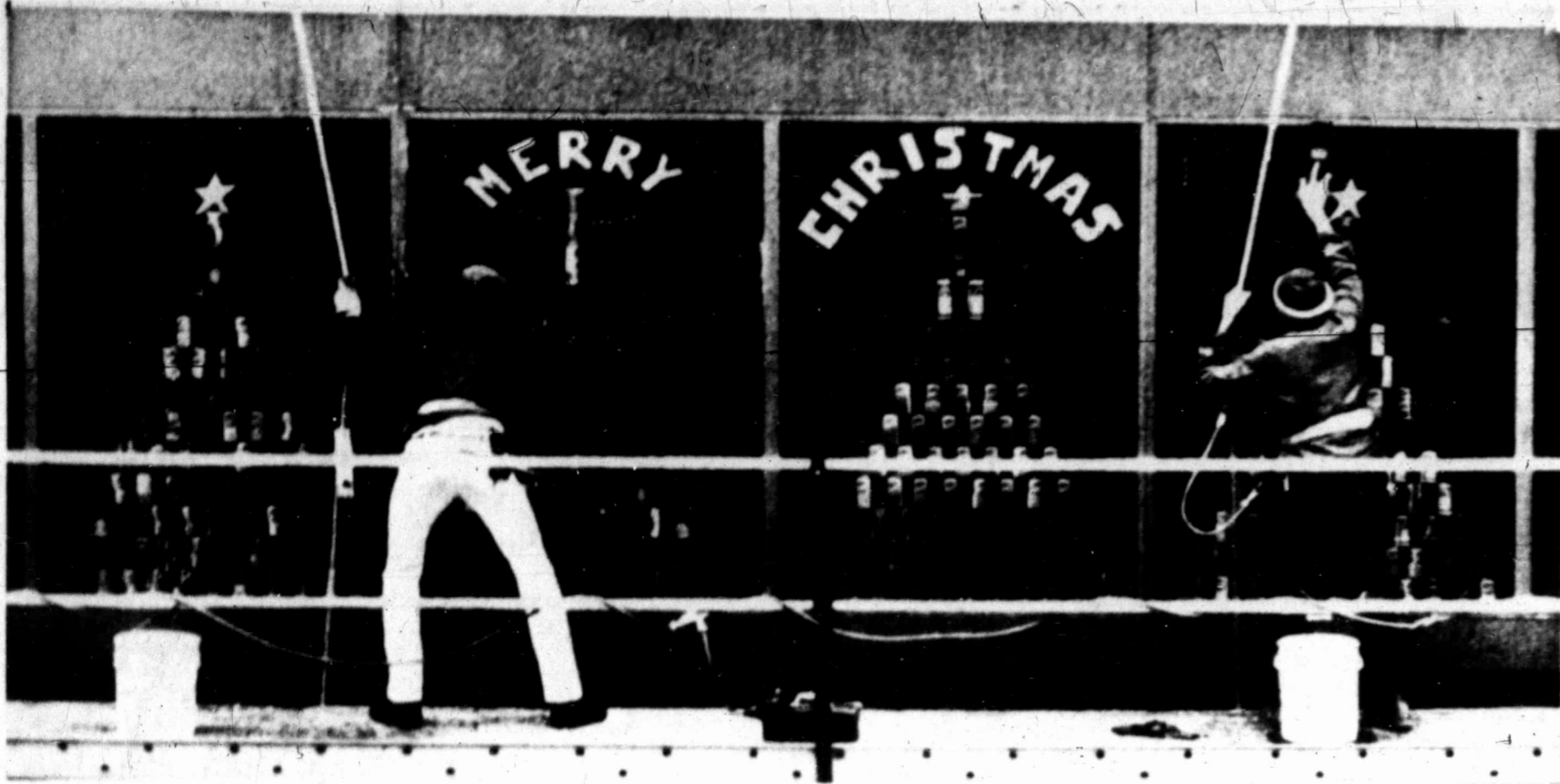
WINDOW WASHERS scrub down windows in a new Washington office building. Construction workers have stacked up soft drink cans in the shape of Christmas trees as decorations.
