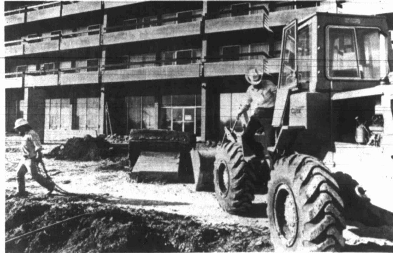
Construction work on Trinity Towers retirement center continues amid increasing costs.
