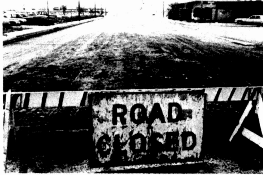
Motorists have noticed several "Road Closed" signs such as this
