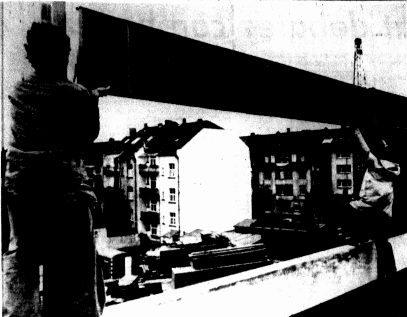
WORKMEN ADD a section of a noise barrier intended to muffle the roar of the autobahn in Frankfurt, Germany, as it passes close to housing.
