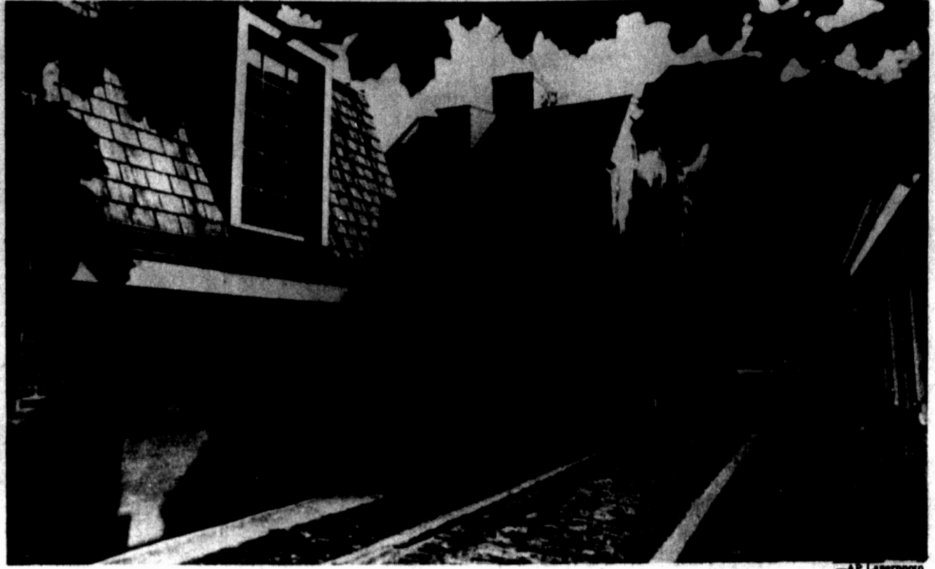
THIS IS THE HOUSE where President Ford plans to stay after his debate with Jimmy Carter tonight. It is a 218-year-old private home in the Society Hill section of Philadelphia. View is from the rear of the house down a cobblestone street.
