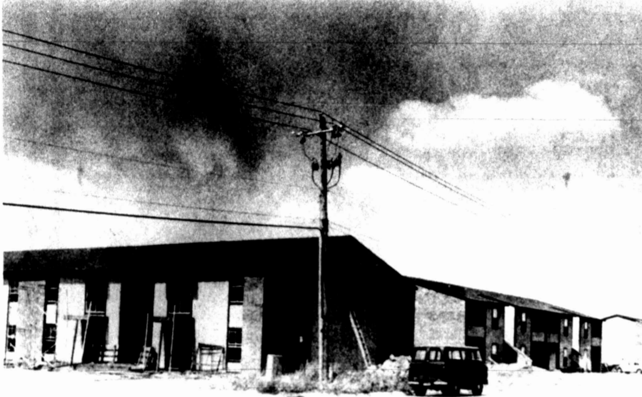
SCHEDULED for completion soon, the Warwick Apartments, 4405 N. Garfield St., are preleasing one, two and three bedroom apartments and efficiencies. The 172-unit complex is developed and constructed by Builders Interest
