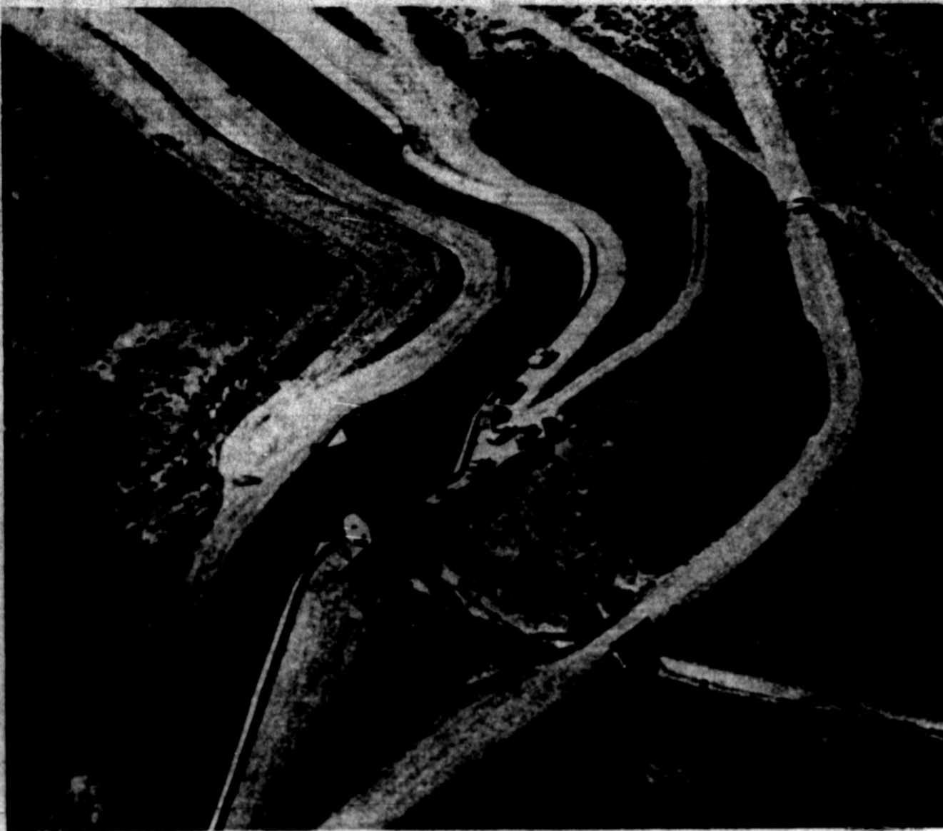
AQUEDUCT WATER, totaling 100 million gallons, flows down a spillway (lower right) and out into the countryside near Lone Pine, Calif., after an explosion blew out a spillway gate in the Alabama Gates building at center of picture. The aqueduct which supplies water to Los Angeles is the dark channel at center of picture.
