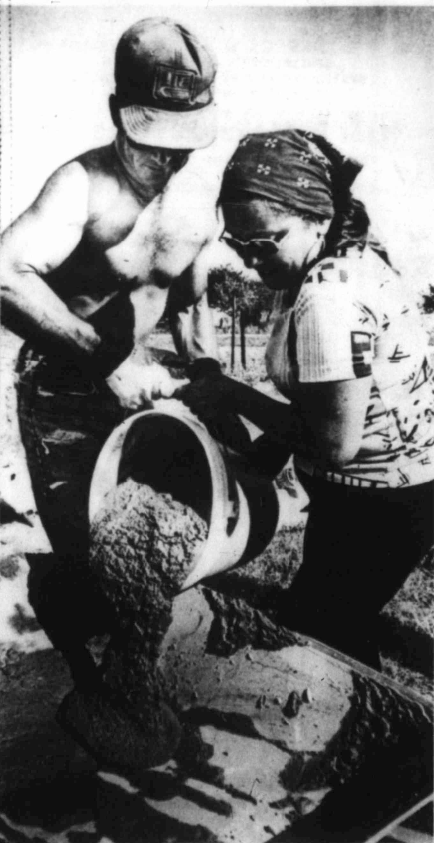
Filling the barrow with mortar.
