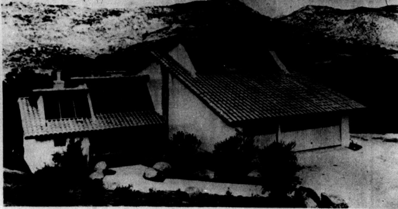
SOLAR PANELS SOAK up the sun's energy to heat this Southern California home. They are incorporated into the roof design as architectural features and furnish the home with hot water as well as heating. —Copley Photo
