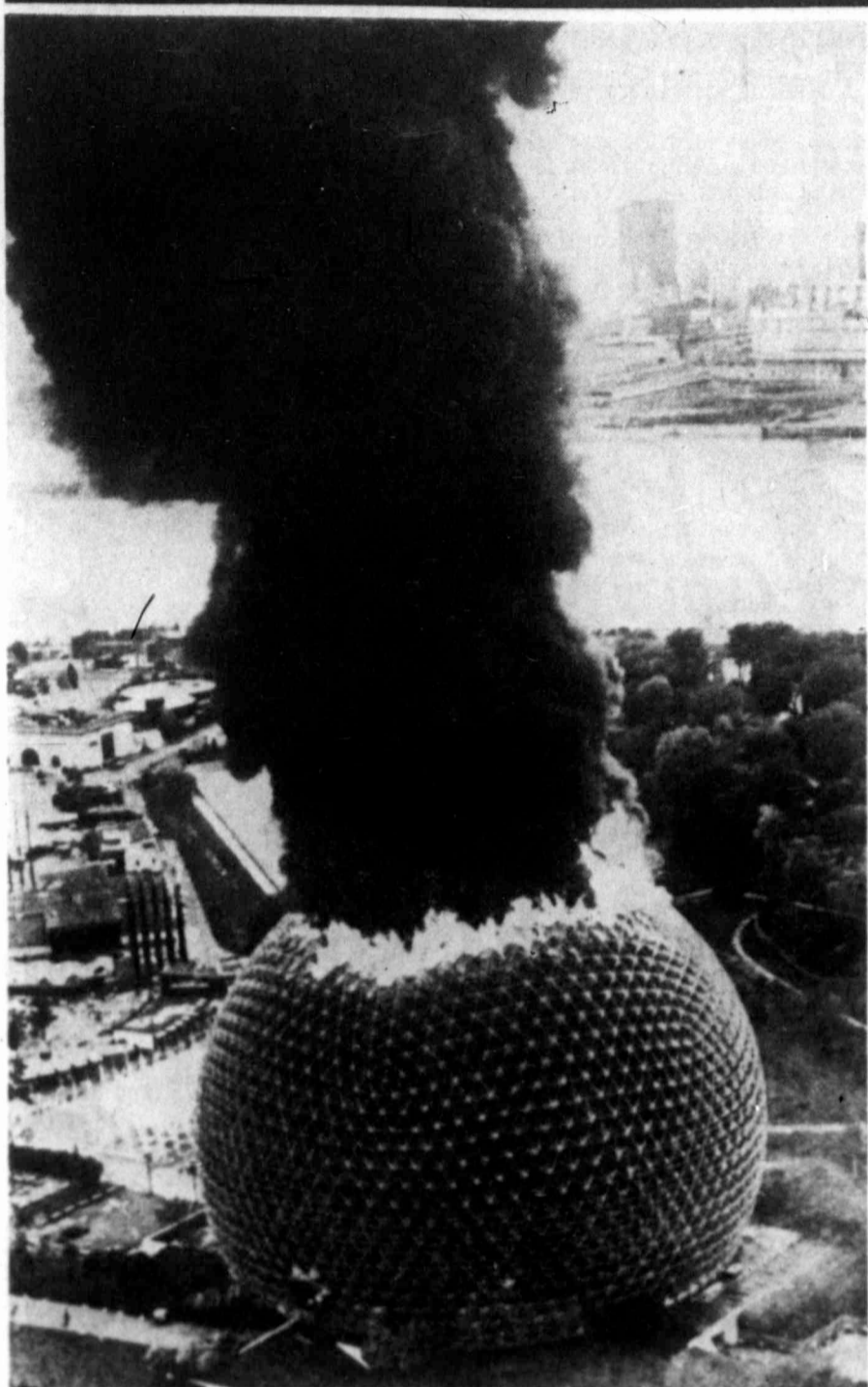
SMOKE POURS from the former U.S. pavillion at the Expo '67 site in Montreal Thursday. The fire destroyed the geodesic dome's acrylic skin, leaving only the aluminum skeleton.
