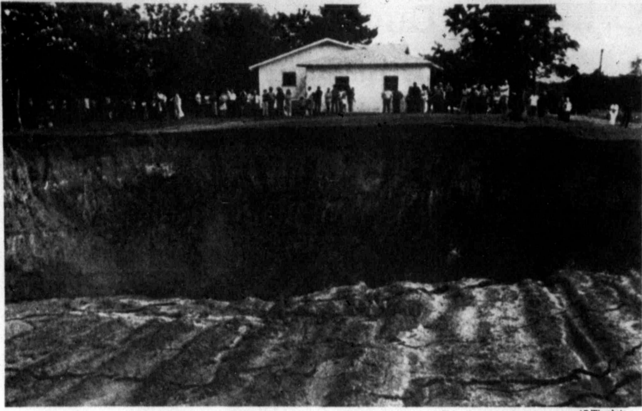
The people of Grand Saline, Texas were in for quite a shock Tuesday as authorities suspect an old brine well collapsed taking out a local road and almost swallowing a house.
