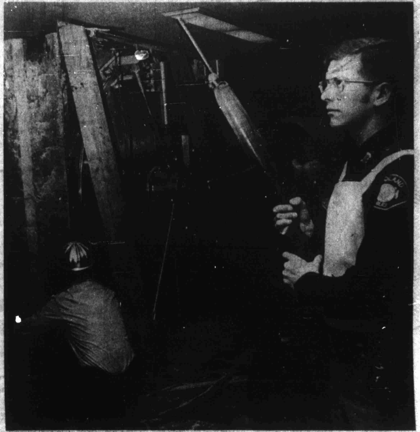
ARMED GUARD Gary Brown, an off-duty Midland policeman, stands at the ready Saturday night as workmen extract the 36,000-pound vault door at The Midland National Bank from a wall. The door will be moved Monday to the bank's new building. Guards armed with sub-machineguns, carbines and shotguns are protecting the open vault. —Staff Photo by Johnny Vines
