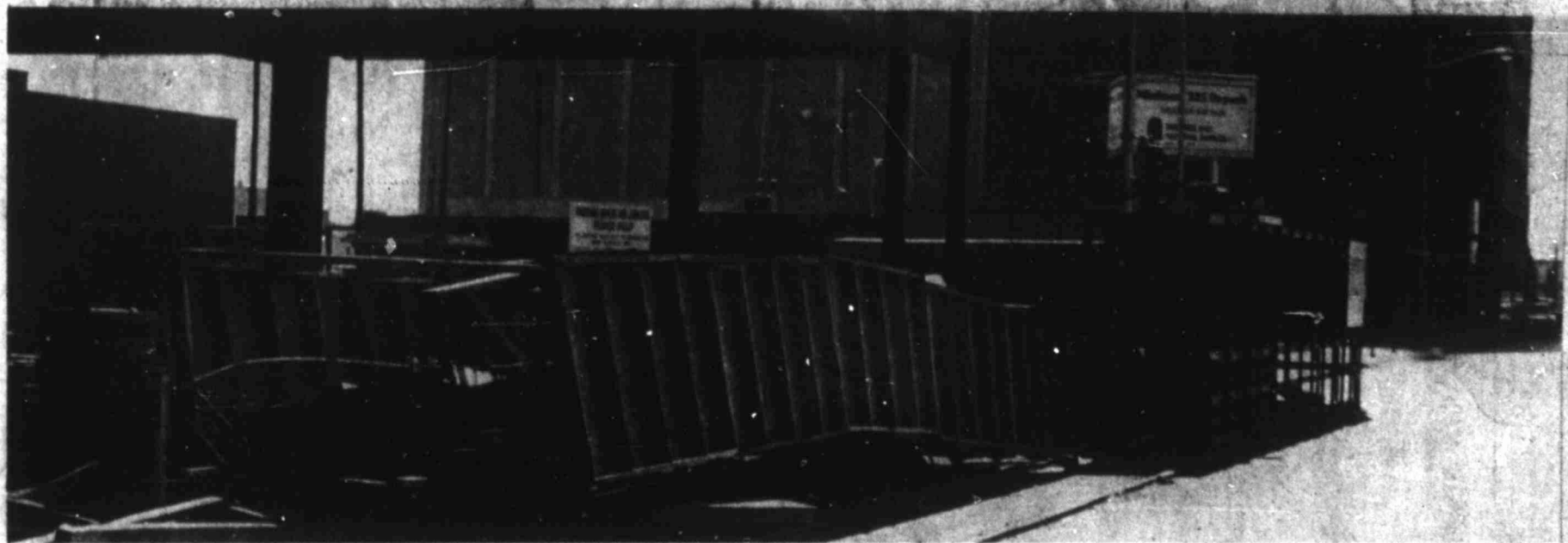
A victim of Saturday morning's harsh winds, the wooden walkway around the Faudree Building construction site lies on its side. —Staff Photo by Charles McCain
