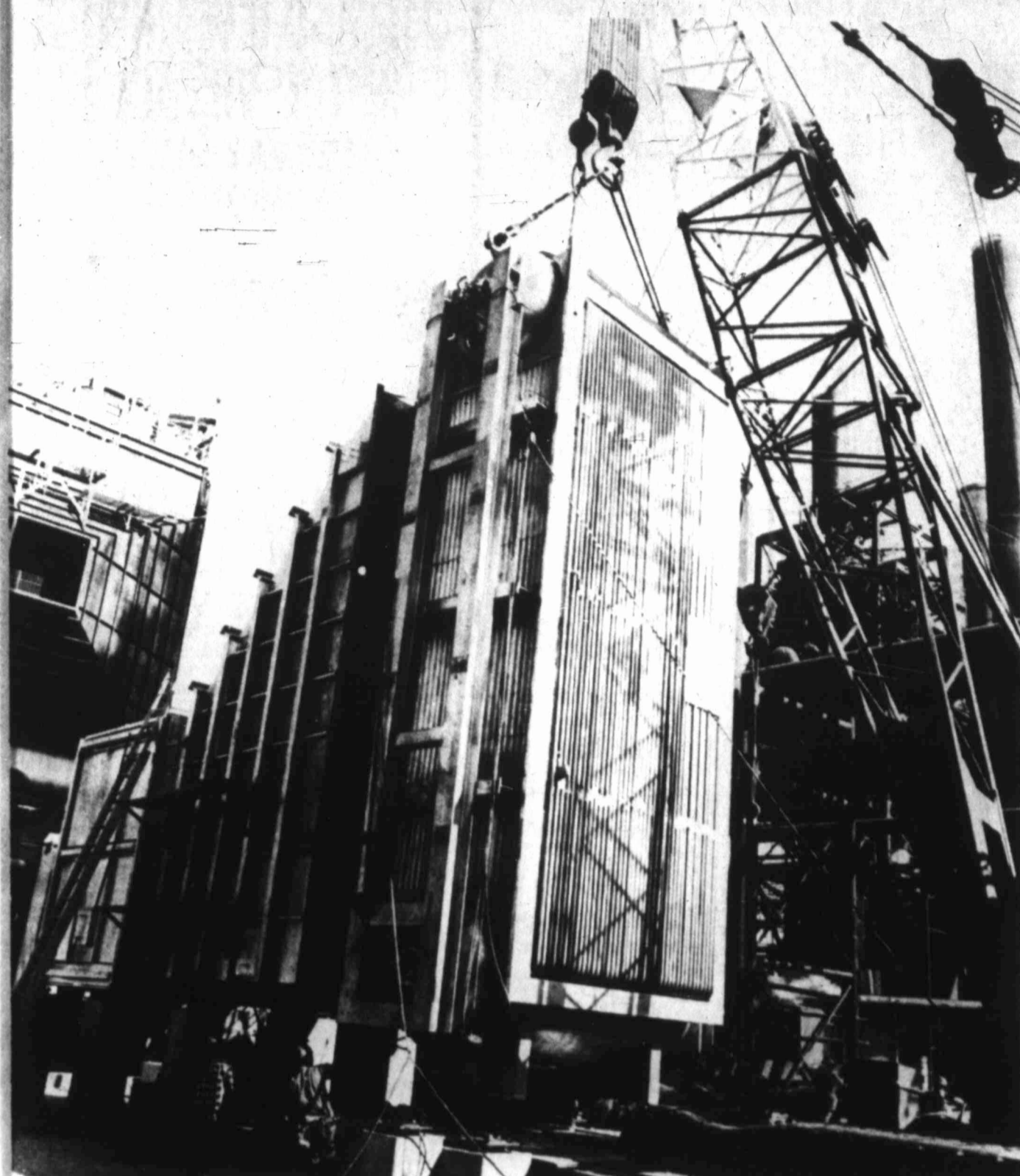
A MASSIVE BOILER, part of a new waste heat recovery unit at Amoco Oil Co.'s Whiting Refinery, Whiting, Ind., is lowered into place. The new unit will substantially reduce atmospheric pollutants and will save energy by producing steam — partially relieving the refinery's power station.
