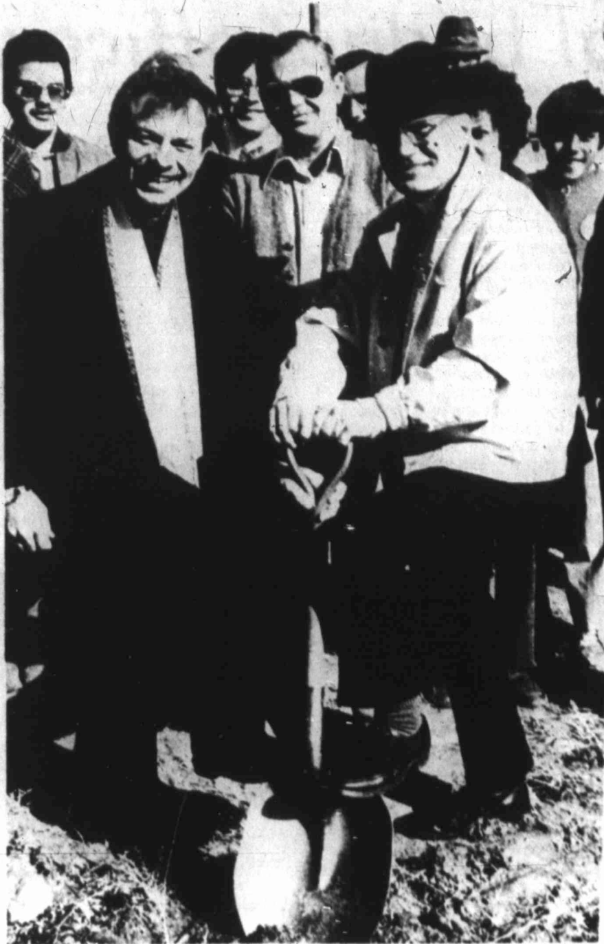
Ground-breaking for a new education building at Our Lady of Guadalupe Catholic Church took place this week. Participating were the Rev. Ron Marlow, left, pastor, and the Rev. Charles Hassenauer, right, associate pastor, along with contractor H. Eugene Abbott, center. Parishioners are in background.
