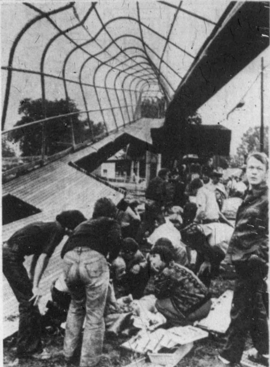
RESCUE WORKERS in Lansing, Mich. Friday attend to injured children beneath the twisted remains of a pedestrian bridge that was knocked down by a crane being used to widen the street below. Six school children were hospitalized after falling from the walkway. (AP Laserphoto)
