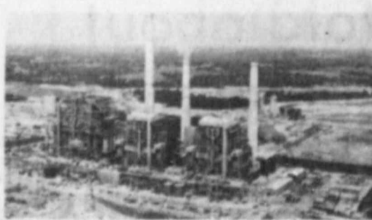
Two lignite coal-fired units are already generating electricity at the Monticello plant near Mt. Pleasant. A third unit is also under construction there.
