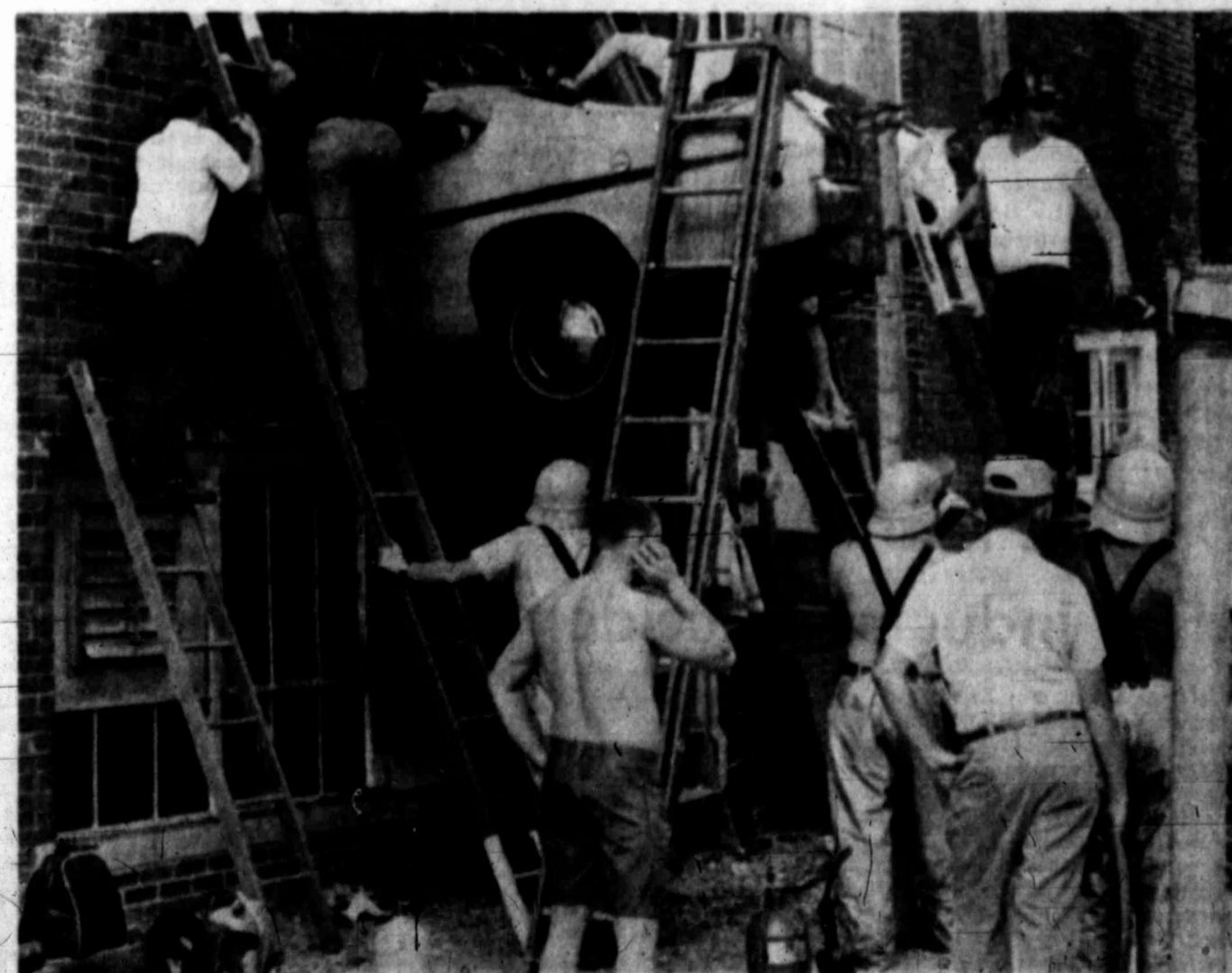
THIS CAR rocketed into College Corner (Ind.) Junior High School after the driver lost control, plowed through the school yard and hit an embankment, police said. Pamela Watkins, 22, of
