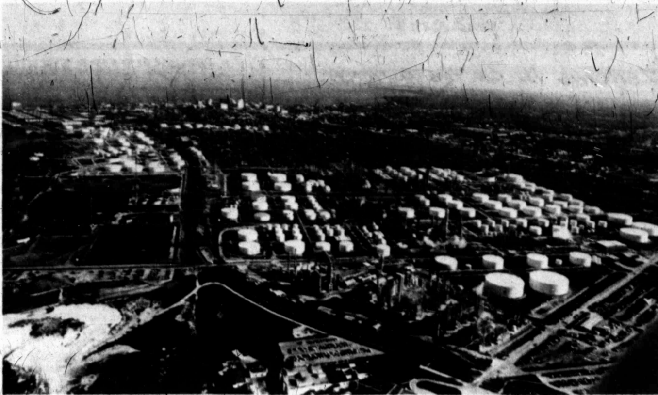
AERIAL VIEW SHOWS Champlin Petroleum Co.'s refinery at Corpus Christi which recently was expanded from 80,000 barrels-per-day capacity to 160,000 barrels. The project was completed at a
