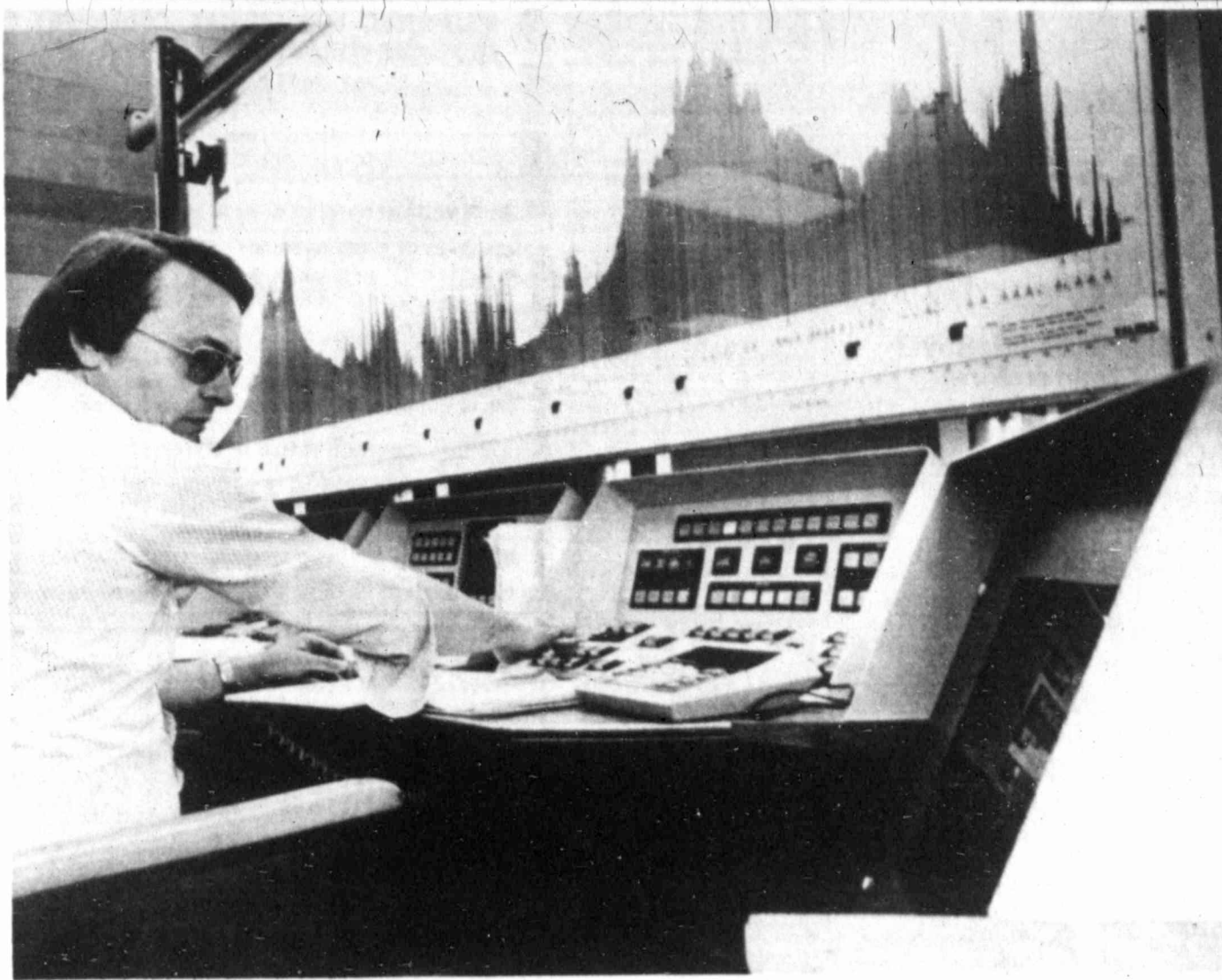
DOUG SHATTUCK SITS at the control panel in the Valdez computer operations control center of the trans-Alaska pipeline as he watches progress of oil fill in the 800-mile-long line. Above the panel is a
