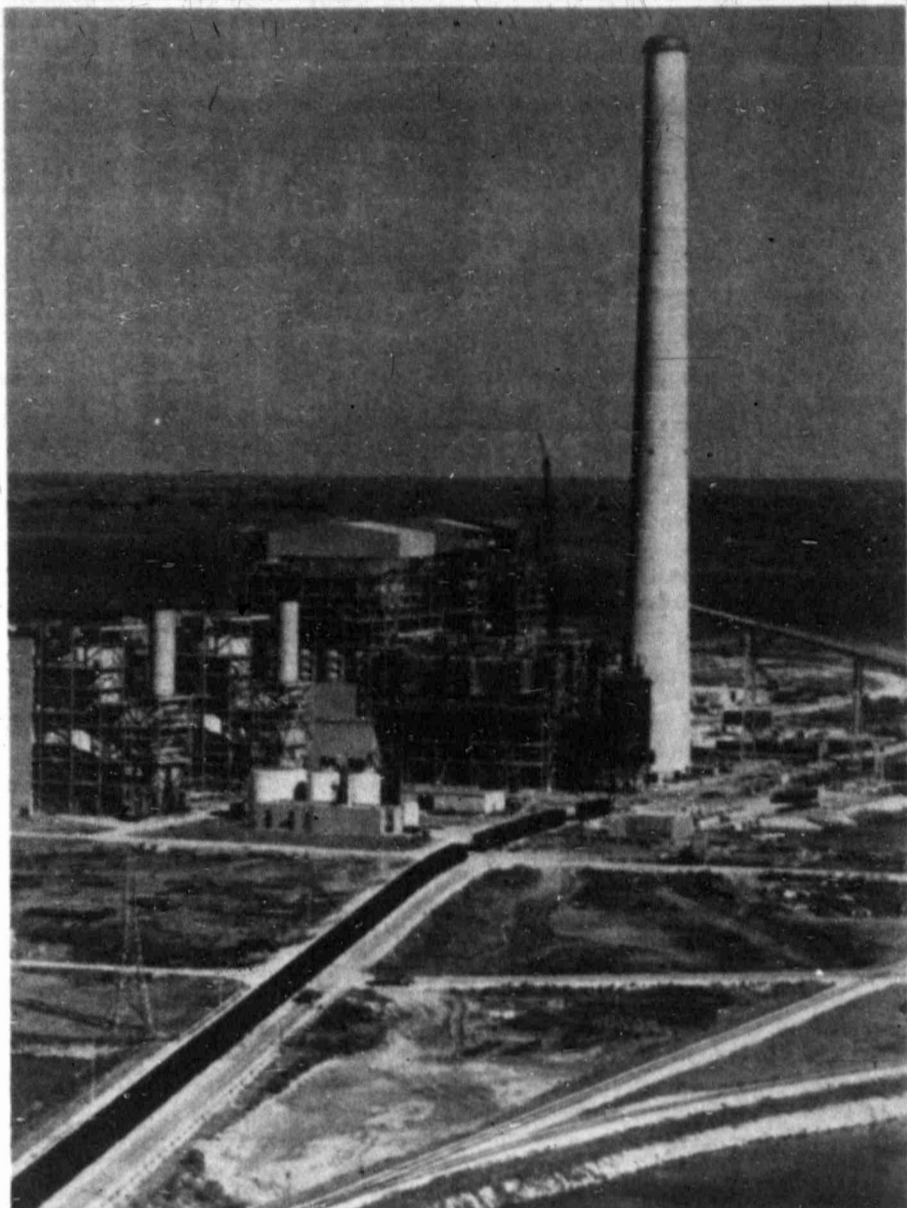
THIS GLEAMING CONCRETE smokestack, towering 700 feet above the rolling countryside, symbolizes San Antonio's determination to curb its addiction to increasingly scarce and expensive gas. The stack is taller than Tower of the Americas, is visible for 20 miles, and is being built at a cost of $326 million. It is part of a coal power plant. (AP Laserphoto)
