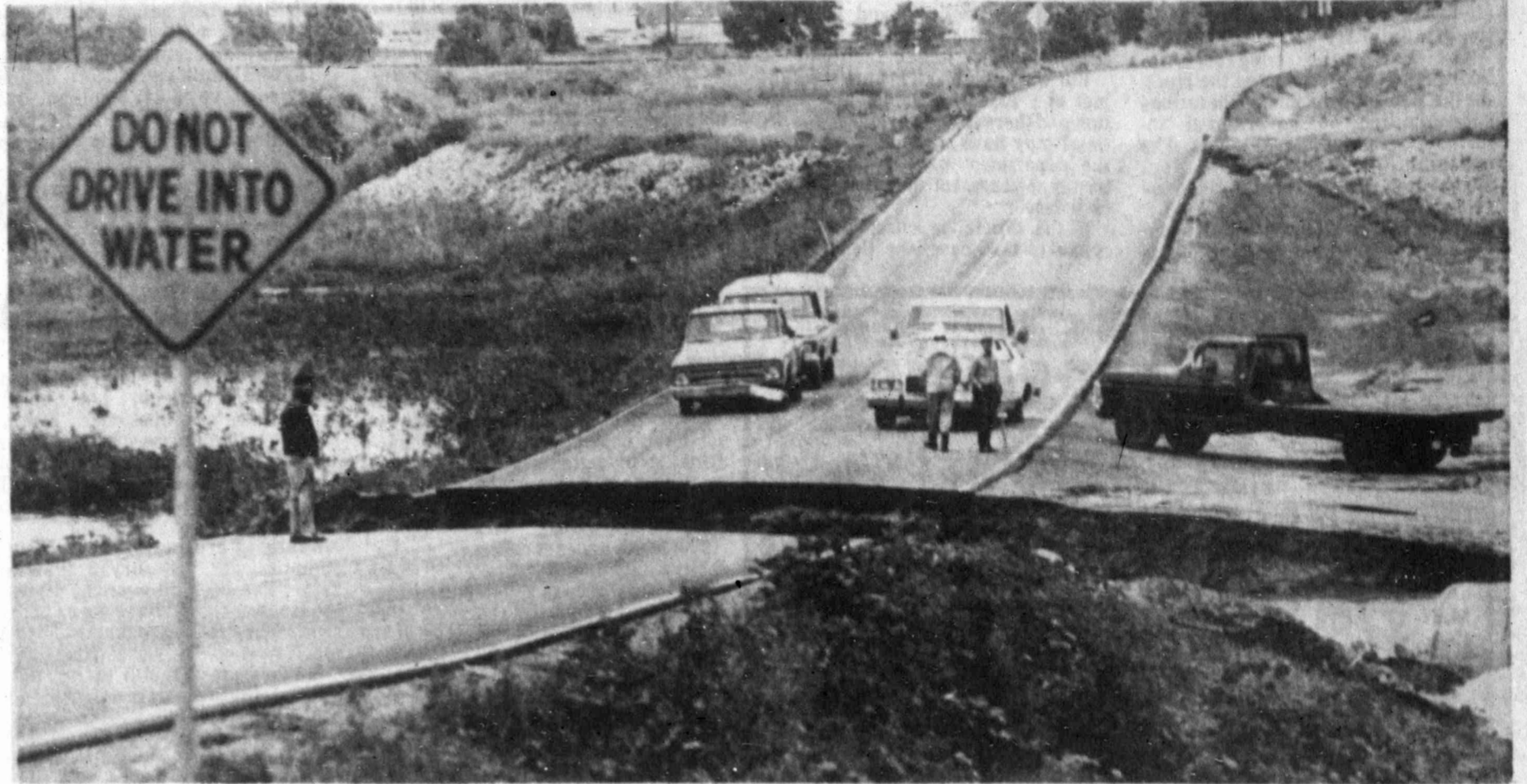
SIGNS HAVE THEIR PLACE on the highways as this one extolling drivers not to go into the water demonstrates at what was a temporary bypass in western Oklahoma City, Okla., before heavy rains damaged it earlier this week. Ironically, the bypass cuts through the North Canadian River while — a nearby bridge is being built. (AP Laserphoto)
