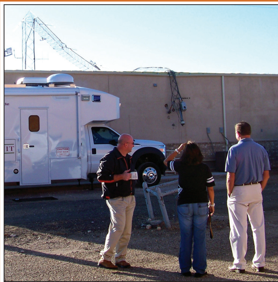
Police Chief Brian Frieda, Mayor Pro Tem Irene Mason and City Manager David Brunson study the damage at the police department after the tower's collapse.
