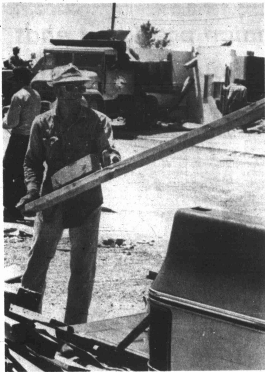
Hutch Reynolds latches onto some salvageable debris 10 days following the tornado that struck Monahans April 19. In the background, city crews continue with clean-up operation.
