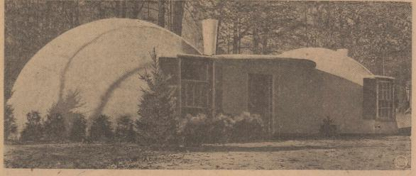
Igloo-like home is result of experiment in rapid building by spraying concrete mixture over large rubberized canvas balloons. RFC's Defense Homes Corporation is constructing the new type houses near Falls Church, Va.
