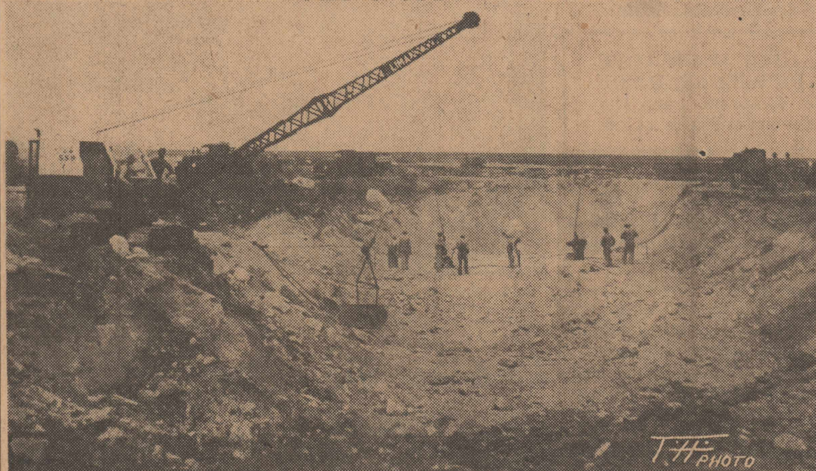
Excavation for gasoline tanks at Sloan Field is nearing completion.
