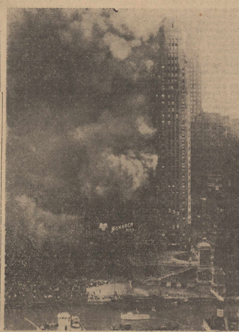
Billows of smoke and flame lick side of Michigan Bvd. skyscraper in Chicago as fire from a freight warehouse (warehouse obscured by smoke but located underneath sign) damages stored merchandise valued in excess of $1,000,000. (NEA Telephoto.)
