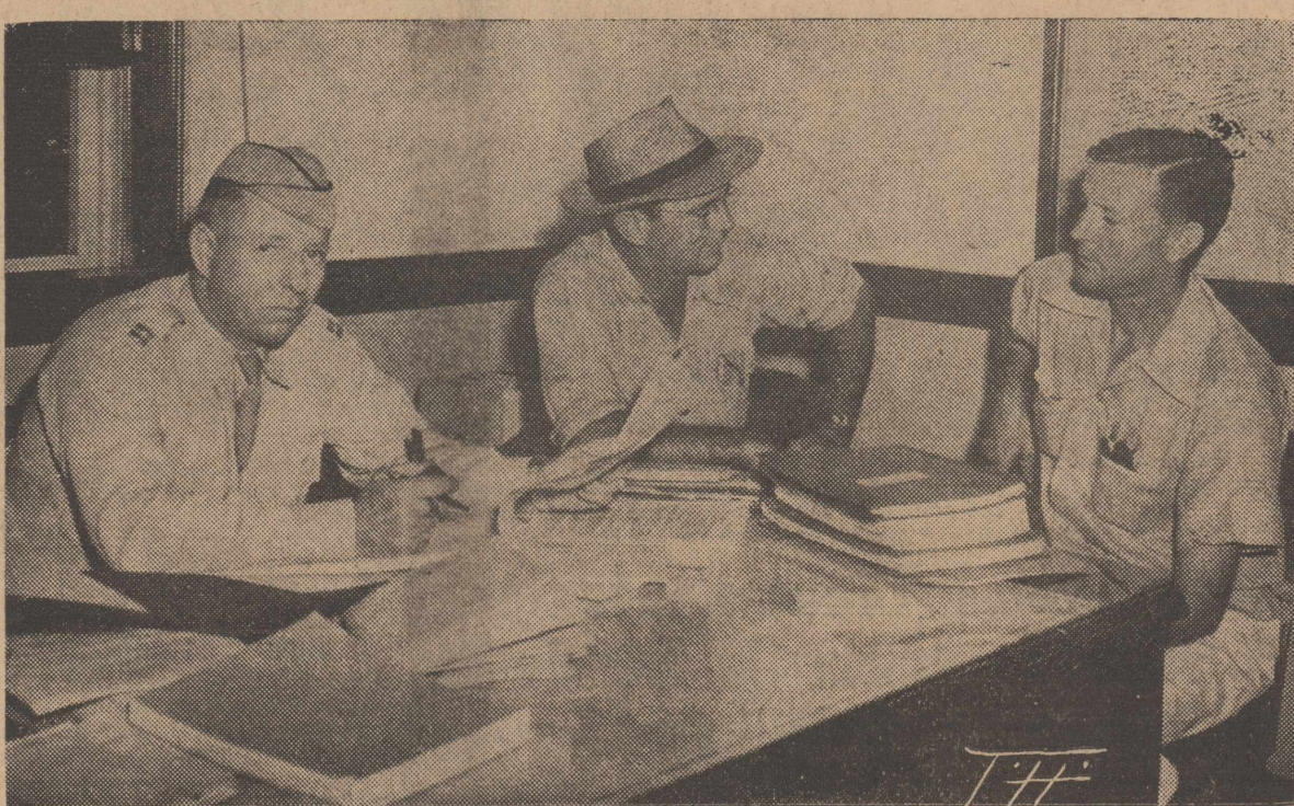
Captain R. J. Harrison of the U. S. Army Engineering Corps, Felix Reeves of Case Brothers and F. M. Reeves and Sons, Inc., general contractors, and R. H. McCulloch, chief engineer, confer on plans for construction of the $5,000,000 Army Air Corps Advanced Twin-Engine and Bombardier Training Center. Captain Harrison is engineer in charge of the construction.
