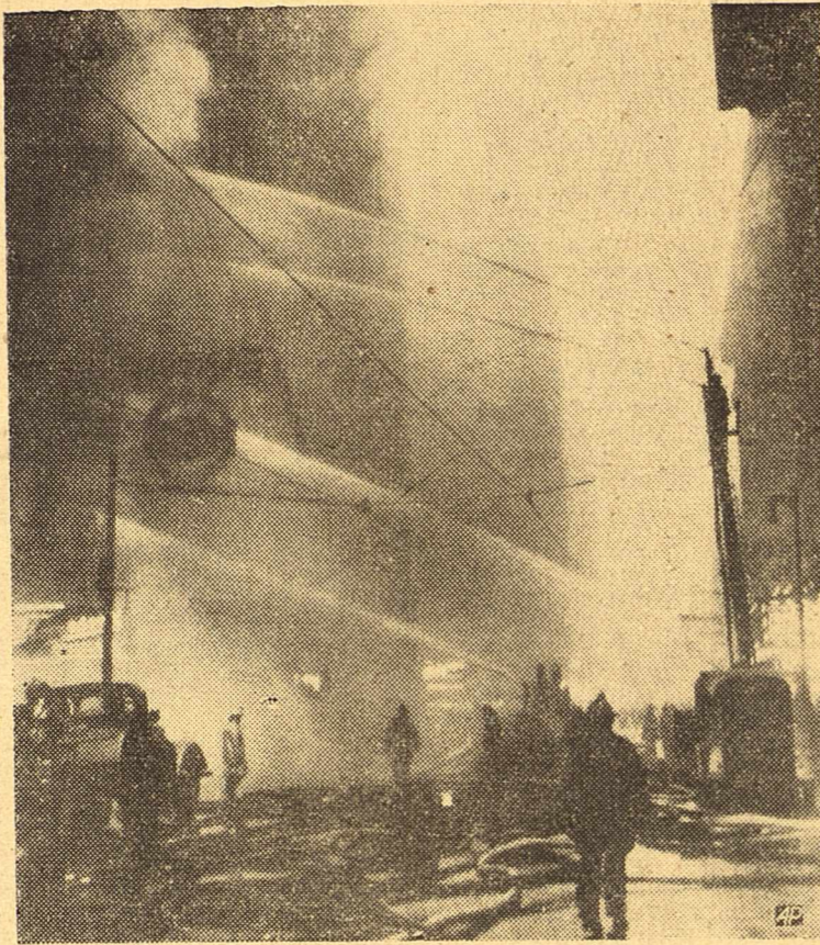
Fire Thursday swept through a four-story restaurant building at 178 West Randolph Street, Chicago, in the northwest party of the Loop. Dense clouds of smoke poured through streets and sparks endangered nearby office buildings.
