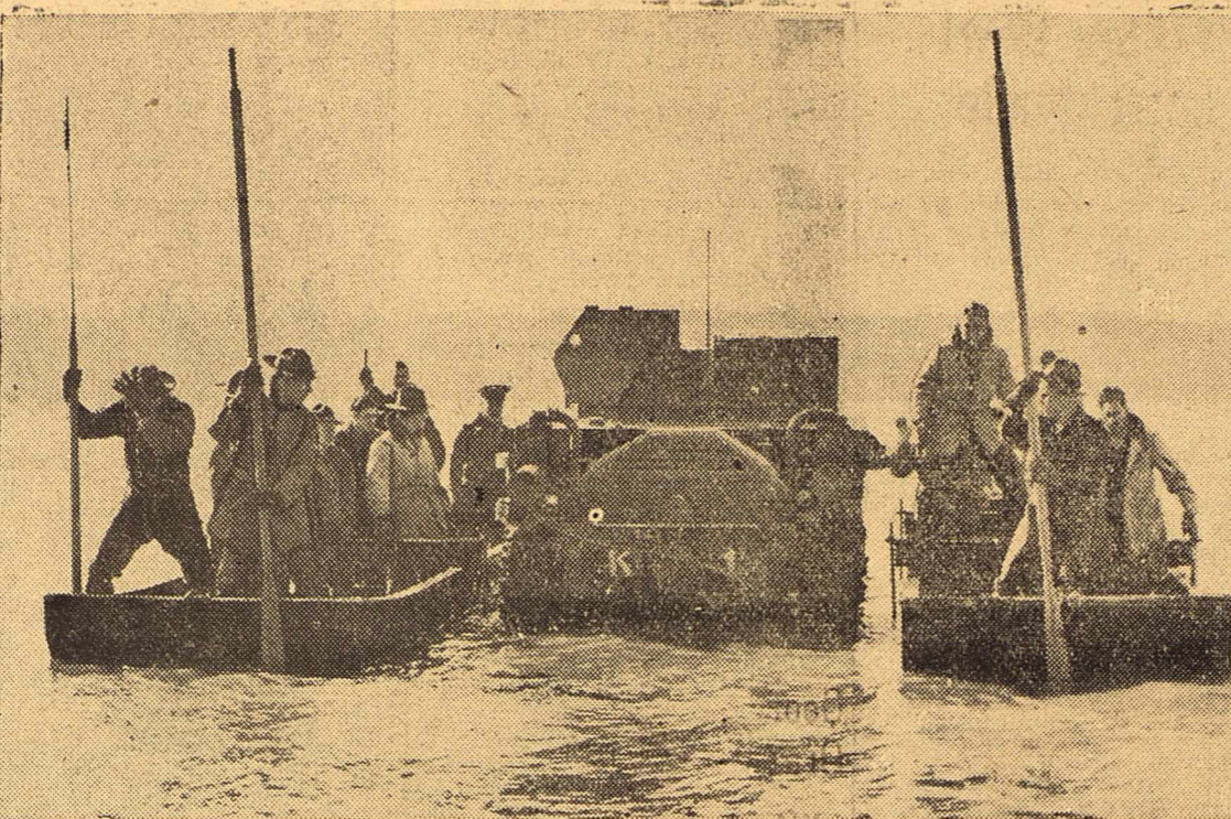
Suppose that a mechanized army comes to a river too wide for quick spanning with pontoon bridges. Why, that's no problem at all, as above photo shows. In a recent demonstration of pontoon ferries, Army engineers from Fort Belvoir, Va., float a medium tank across the river, supporting it with those pontoons at either side.
