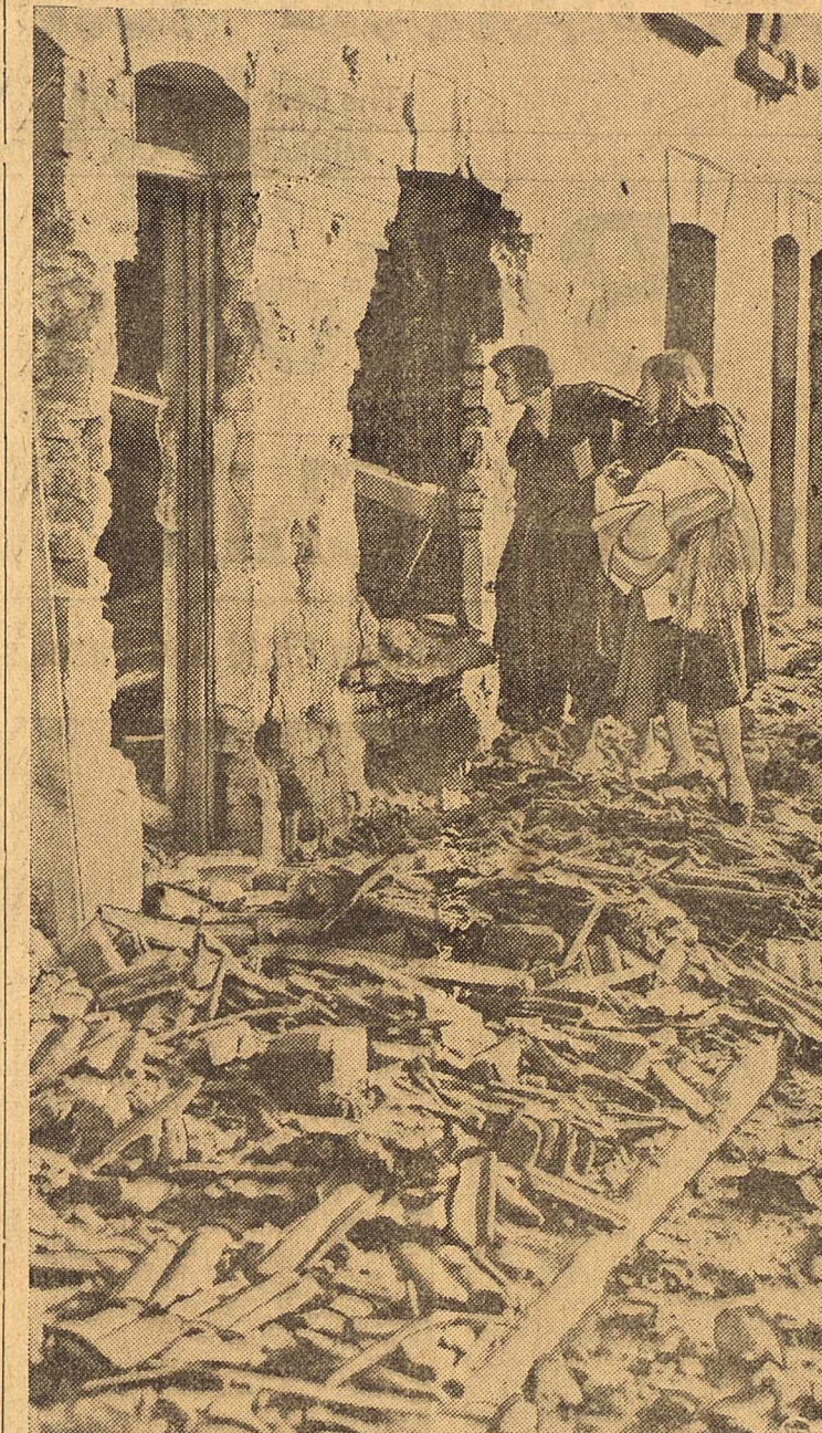
Fleeing down a wreckage-littered street in London's working-class quarter, these two girls, arms laden with hurriedly-snatched blankets and clothes, pause to peer through gaping hole torn in a tenement house by German bombs. Photo passed by British censor.
