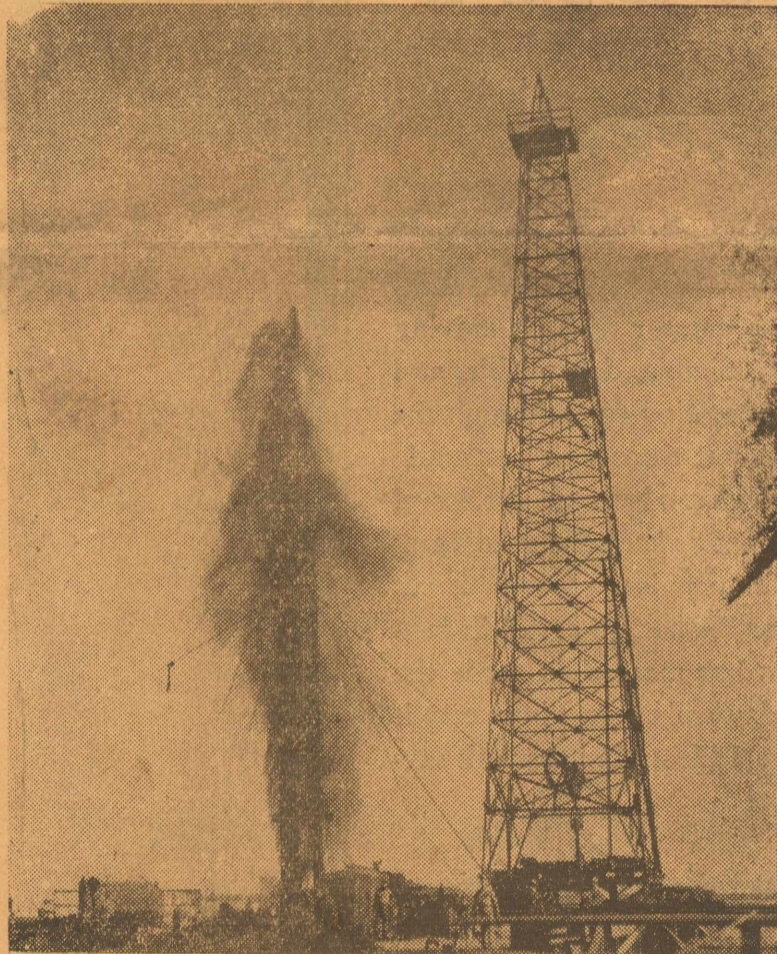
Above is shown C. A. Everts of Dallas No. 1 John M. Gist, new well in the Foster pool of Ector county, heading oil after nitro shot.
