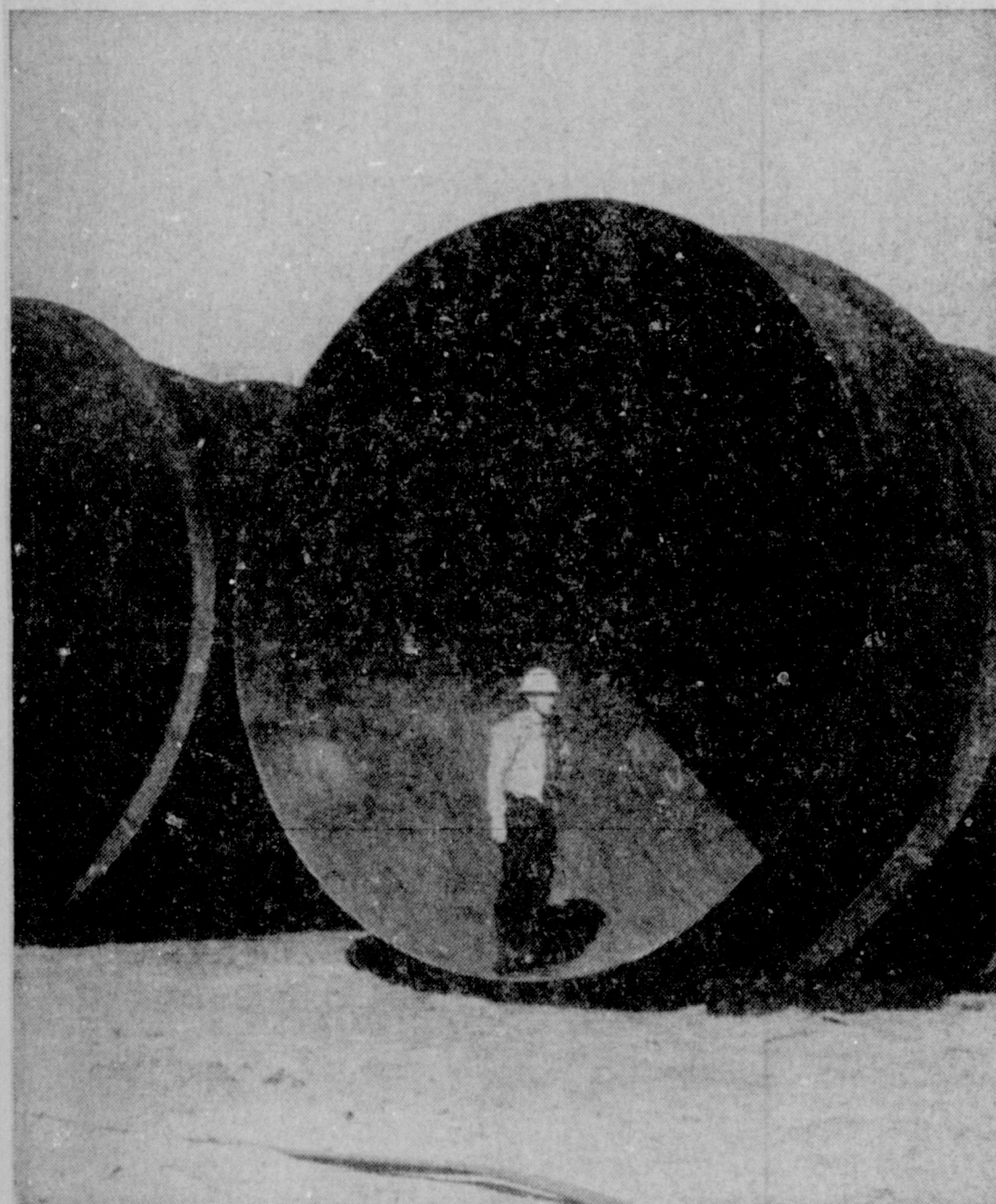
Flood Control Pipes Dwarf Man
