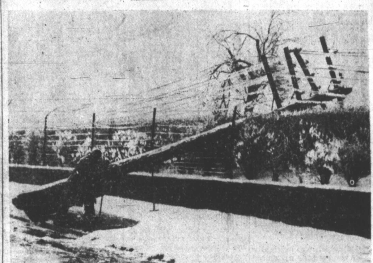
Rain, sleet and snow combined to cause a million dollar damage in snapped power lines, interrupted communication lines and broken-down trees along the eastern seaboard. Shown above is a typical scene near Rutherford, N. J., where the weight of ice-covered lines caused this and many other poles to fall.
