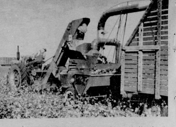
'GREEN BOLL' SEPARATOR - Here's cotton receipts considerably. After the machine which separates the green bolls able. (Extension Service Photo) from mature cotton, is calculated to up
