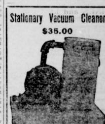
Driven by GASOLINE ENGINE or Motor One of the Best on the Market. Place in Cellar or Outer Building and Pipe to Each Floor Where the Hose Is
