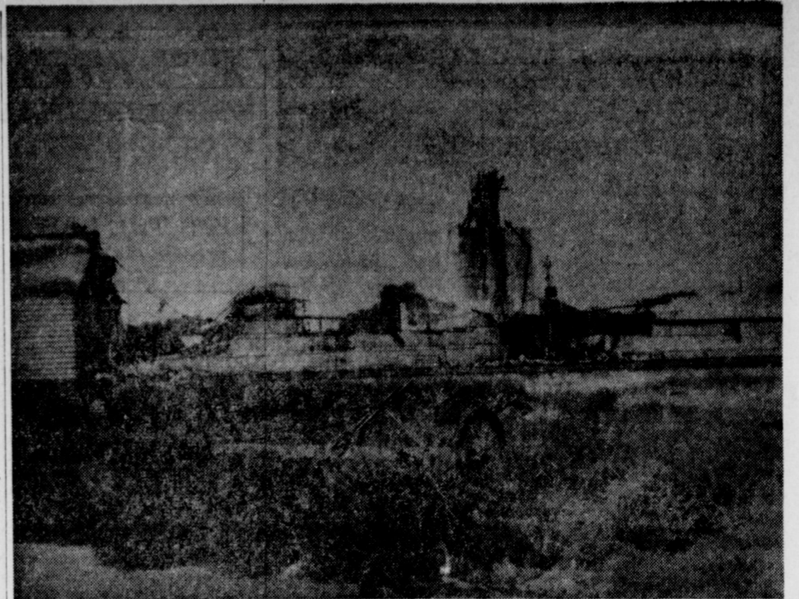
REBUILDS — Muleshoe Elevator Co., hit by a $155,000 fire a week ago, is already in the process of rebuilding. The center section of the big elevator was razed and 17 cars of grain were destroyed in a blaze which raged out of control for more than a hour. This shows the ruins the next morning. Firemen were able to save adjoining sections of the plant. (Journal Photo and Engraving)
